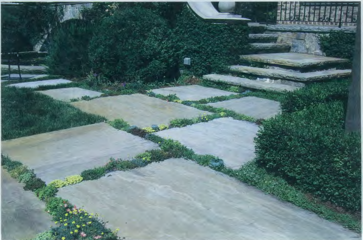
Slight gaps left between the large slabs of rustic Yorkstone pavers were planted with a variety of sedums.
